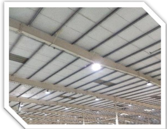
Lighting effect after the replacement
